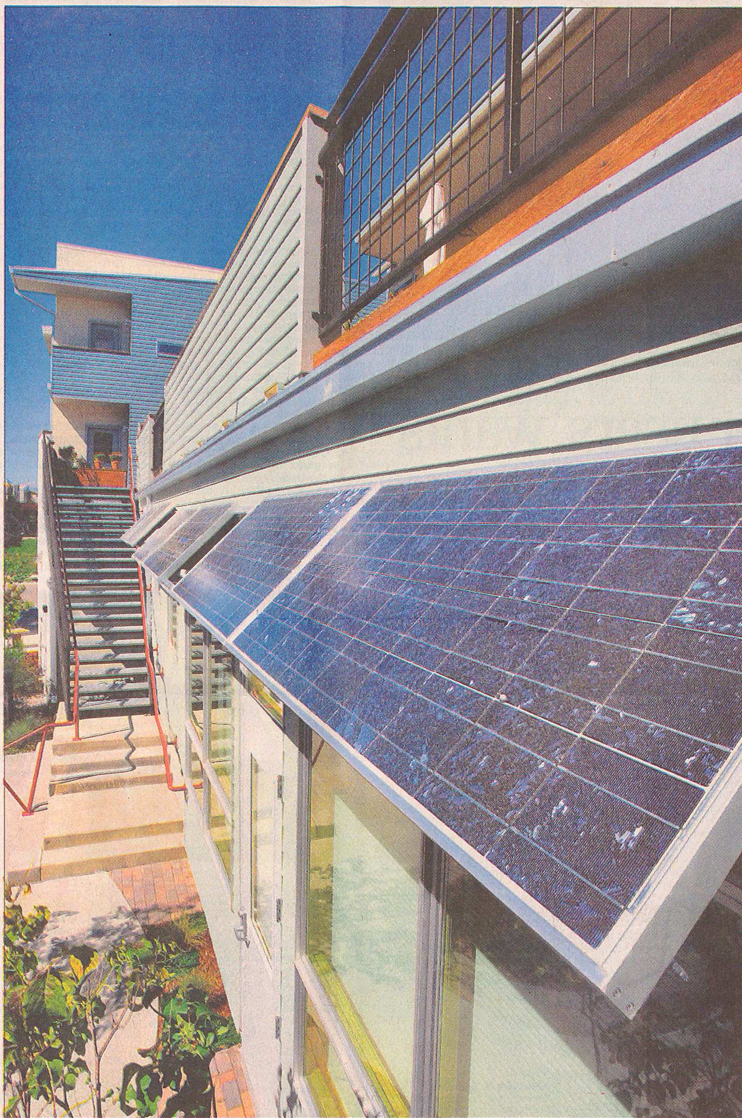
Solar panels serve as permanent awnings above south-facing windows. The panels from Sun Electric Systems also generate
