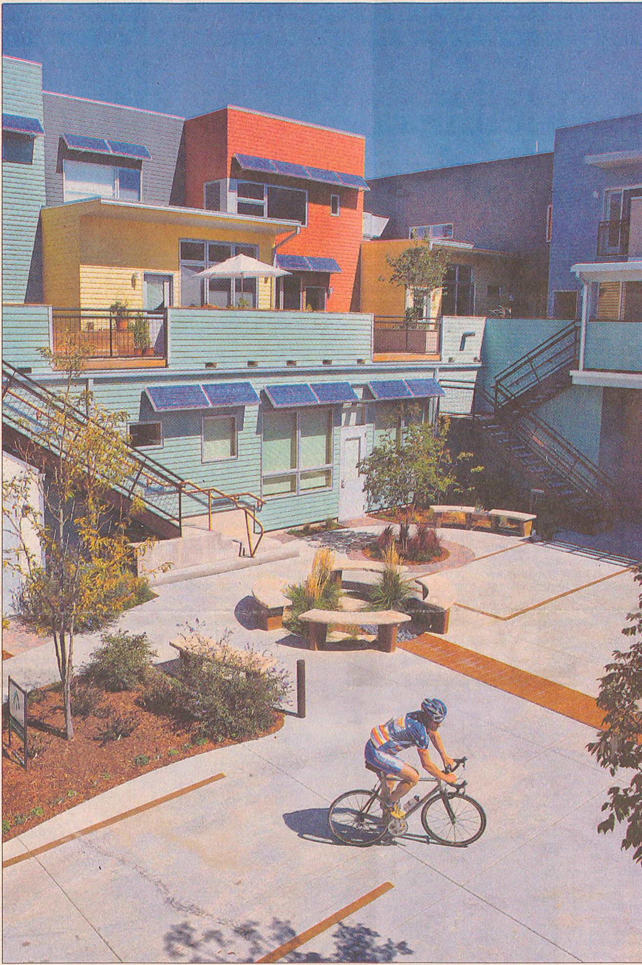
Stucco-covered peaks hold solar panels up to the sun. The units provide hot water for everything from in-floor heating to bathing at Solar Village Prospect.
